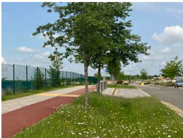
Figure 84; Tree planting, with a swale
